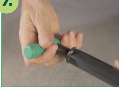
In preparation for installing the pipe onto the fitting assembly, reaming is required. Insert reamer into pipe end. Turn the reaming tool 3-5 rotations with enough force to cut a bevel into the pipe end. Remove the reamer and inspect pipe end. Remove shavings if present.
