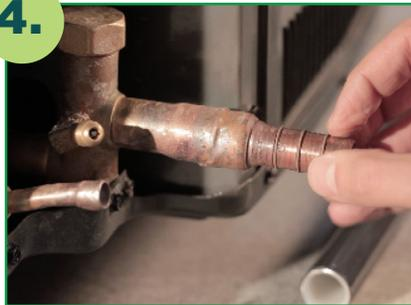
Carefully roll the o-rings into the recessed grooves on the fitting body. Start with the first groove and work towards the back of the fitting as the o-rings will roll over the rings that have been already seated in the grooves. Lightly spinning the o-rings will ensure they are not twisted and are properly in place.
