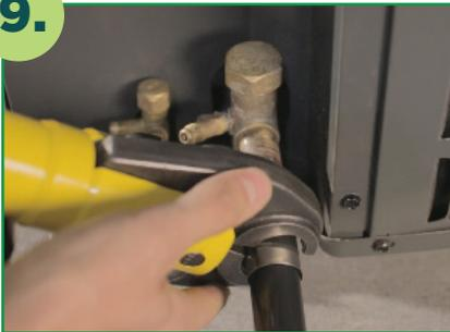
Ensure proper sized crimping head is selected. Open jaws and place over stainless steel crimp sleeve, positioning tightly against the plastic isolation collar. Keeping the tool perpendicular to the fitting and properly positioned, complete crimp using manual or power crimping tools. Ensure that the jaws of the crimping tool come together completely.
