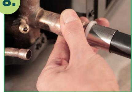
Push pipe onto fitting and into sleeve until pipe is visible through the inspection windows in the stainless steel sleeve.
