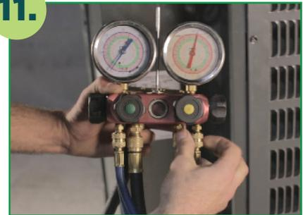
After completion of the crimp, proper pressure testing procedures should be followed to check for leaks. As per ASHRAE guidelines, a proper vacuum should be performed on the system to ensure system is free of moisture and contaminants.
