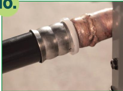
Remove tool from crimped connection and inspect for three circumferential indentations on the stainless crimping sleeve.
