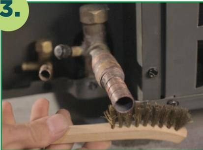
Visually inspect completed brazed connection for any potential leak points
